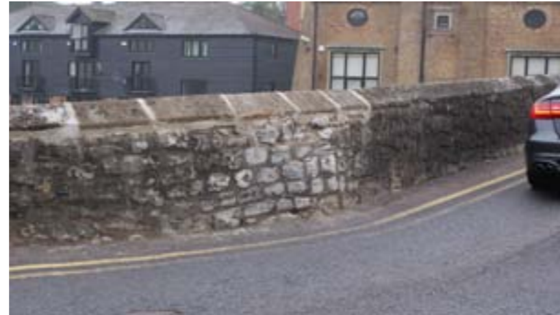
Above and Below: Repaired damage to north and south western corners of bridge. Example of how new stonework is unsympathetic to historical masonry.
