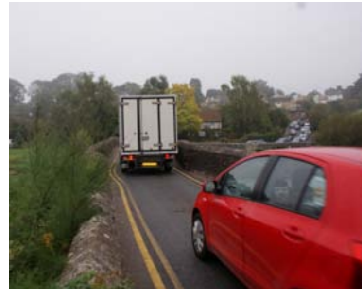
Below: An image of another small lorry crossing the bridge highlights the significant lack of room available to pedestrians when over sized vehicles cross
