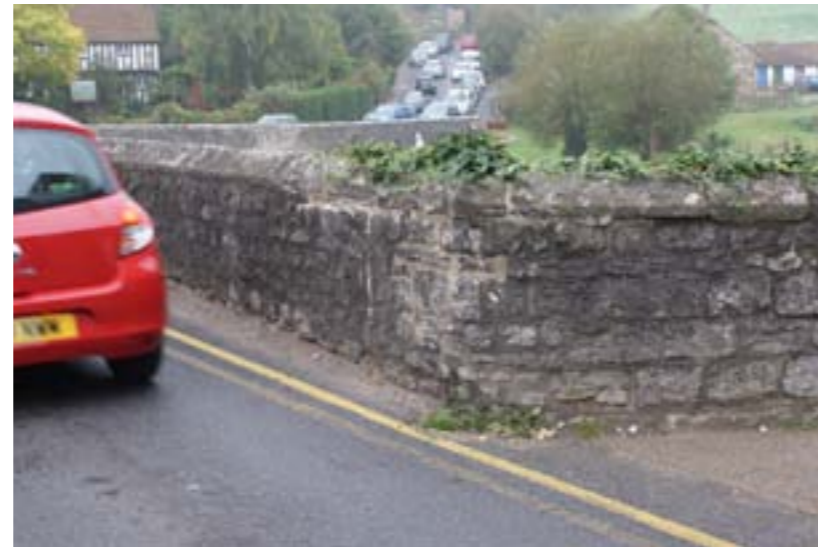
Above and Below: Repaired damage to north and south western corners of bridge. Example of how new stonework is unsympathetic to historical masonry.
